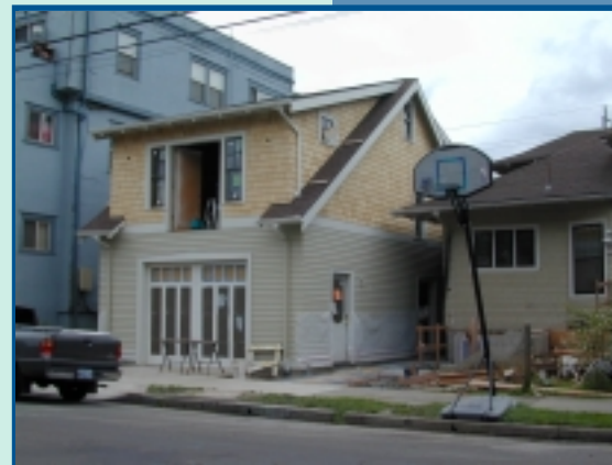
Irvington: under construction
